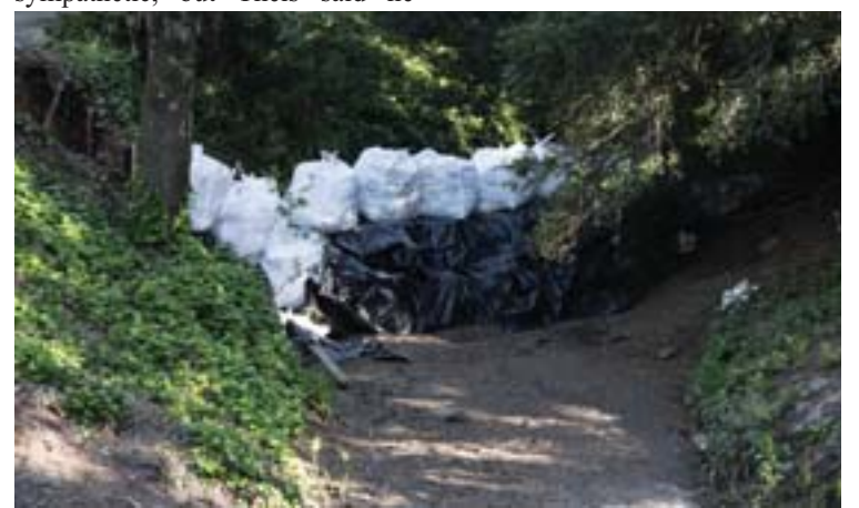
A temporary dam and the dewatered creek bed.
